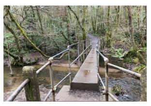
Our proposal for the works would be to remove the existing footbridge, excavate behind existing retaining walls and remove / or include within new interlock concrete block retaining walls either side of the river.
