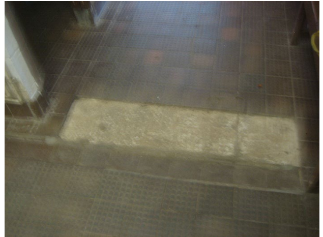
Damaged tile floor in the front right changing room.
