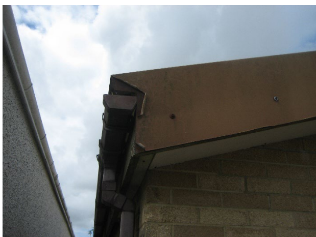
Vergeboarding and soffits on both the left and right hand sides of the property were in need of repair or replacement.
