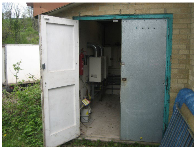
Timber doors with metal cladding giving access to the plant room require replacement.
