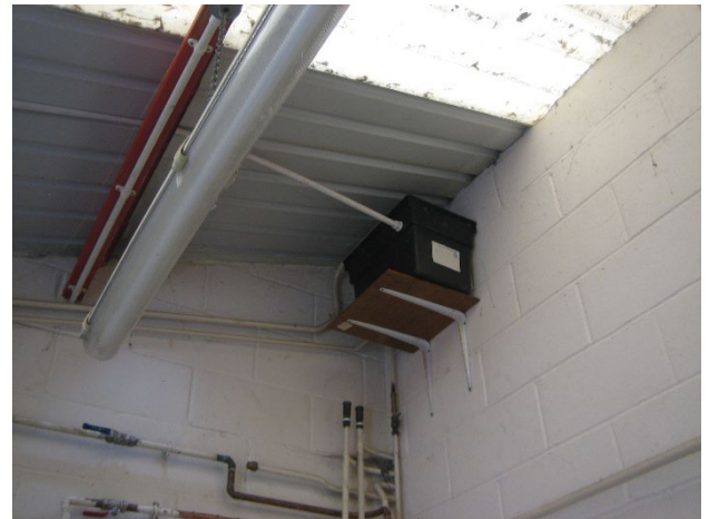
Central heating header tank in the Boiler Room.
