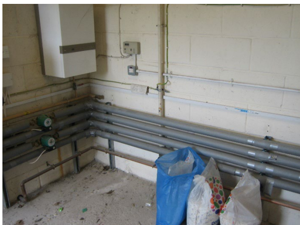
Concrete floor and insulated pipework in the Plant Room.
