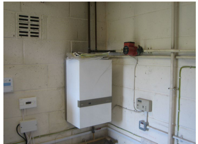
Gas boiler in the Boiler Room.
