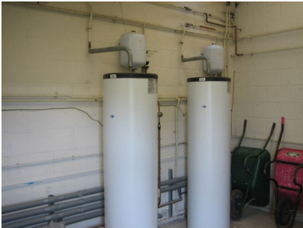
Hot water units in the Boiler Room.
