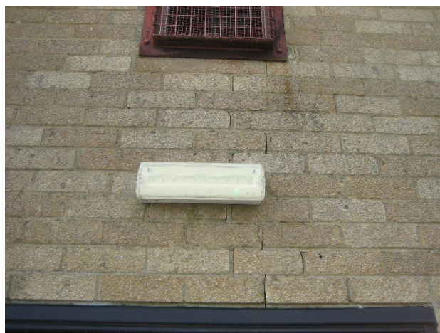
Minor hairline cracking in the brickwork above the right hand door.
