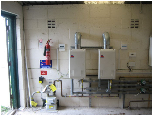
Andrews water heaters on the rear wall of the Boiler Room.
