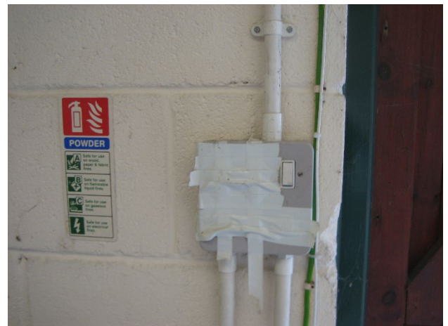
Light switch which requires repairing in the Plant Room
