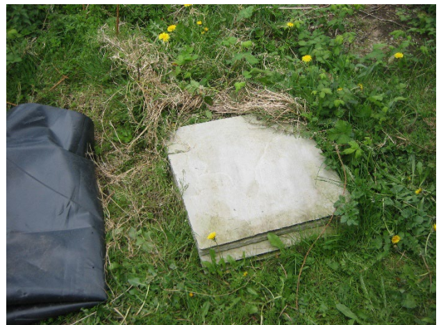
Manhole cover which requires replacement adjacent to the Boiler Room door.
