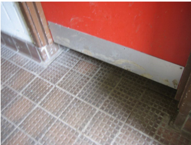
Gaps were noted at the bottom of the door to aid ventilation.
