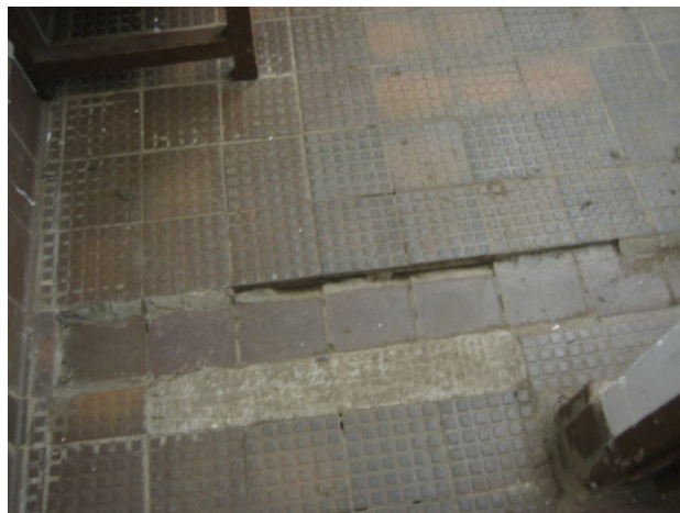
Damaged tiling forming the floor in Changing Room 1 requires repair.
