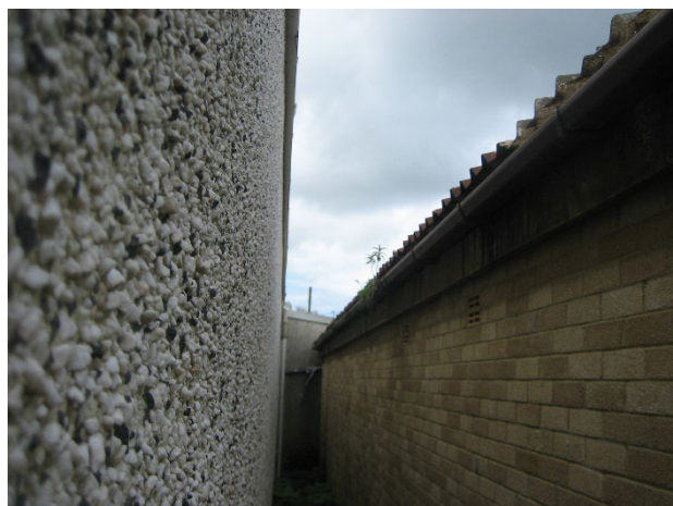
uPVC gutters and fascias on the front of the property were in need of repair and the gutters require clearing.
