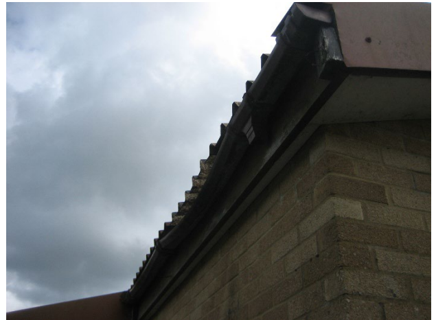
Damaged guttering on the rear left hand side of the property should be replaced along with the fascias.
