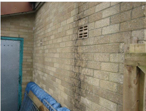
Staining on the wall as a result of the damaged guttering.
