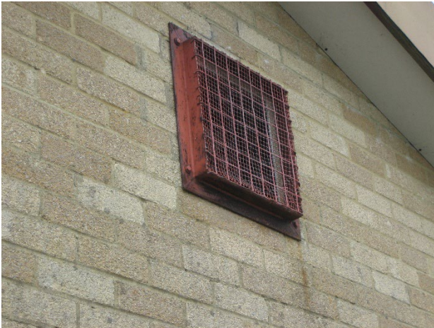
Metal vent grille above the right hand door requires repainting.
