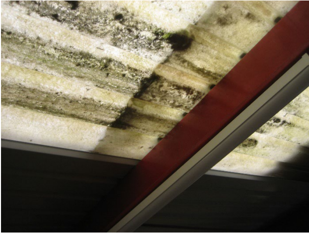
Clear panels set into the roof require cleaning.
