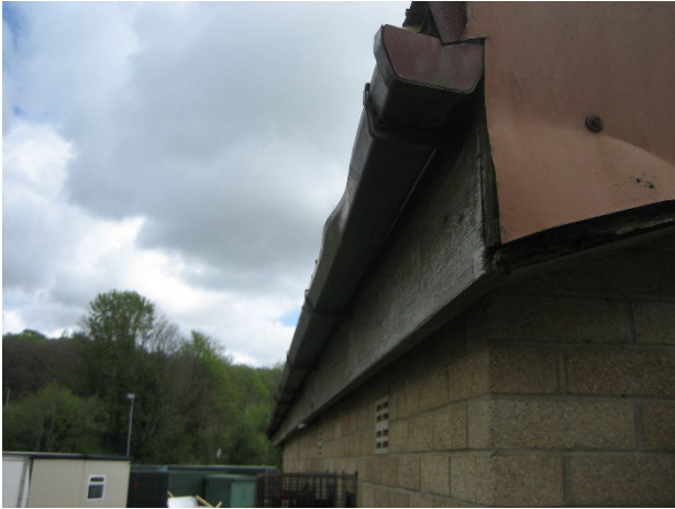
Fascias and soffits on the rear of the property require repair or replacement.
