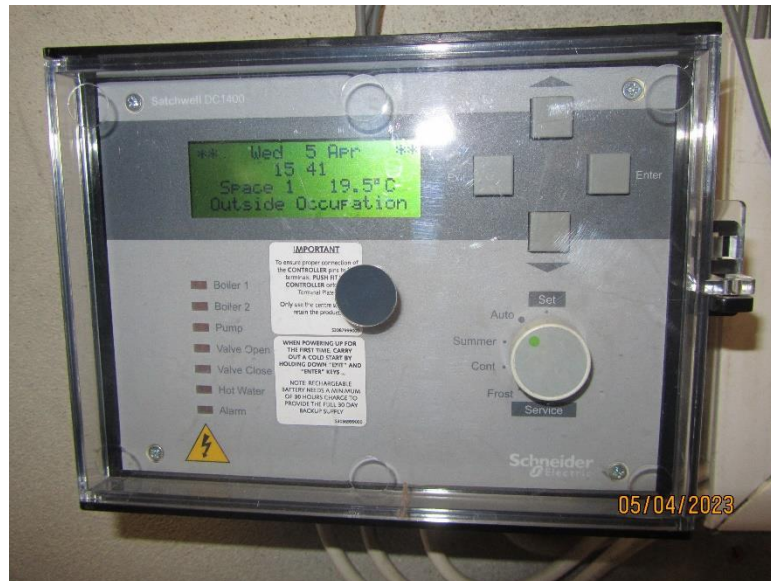
Figure 14 Existing main control panel for heating and hot water
