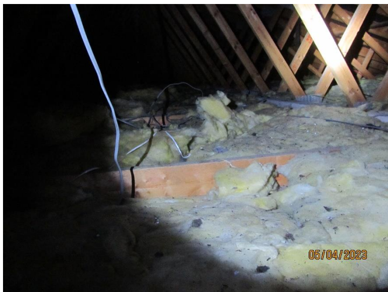
Figure 10 Insulation is not consistent in its application
