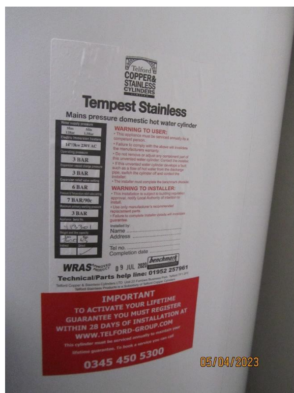
Figure 16 Specifications from one of the hot water tanks in new changing rooms
