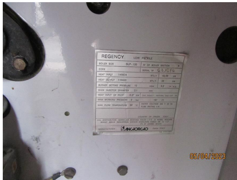
Figure 12 Main boiler specifications
