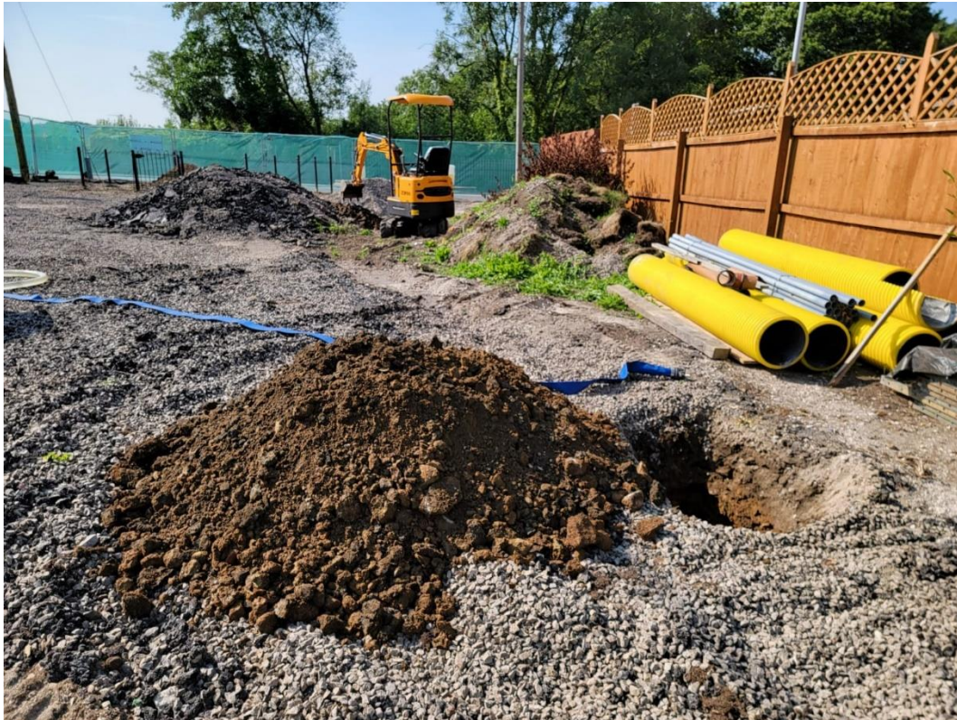
Picture 1 – Test Pit 1 location
