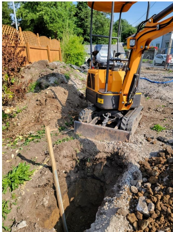
Picture 2 – Test Pit 2 Location
