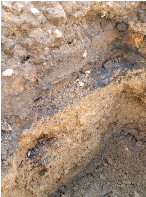
Picture 3 – Test Pit 2 Ground Strata's
