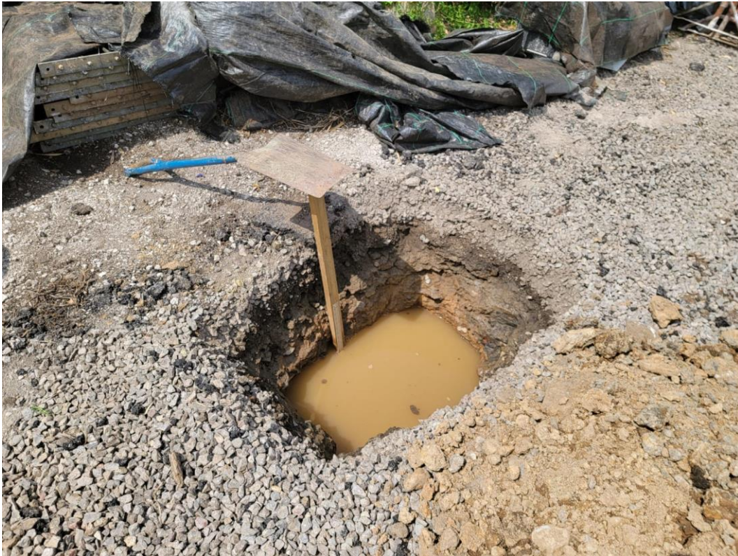
Picture 5 – Test Pit, test 1
