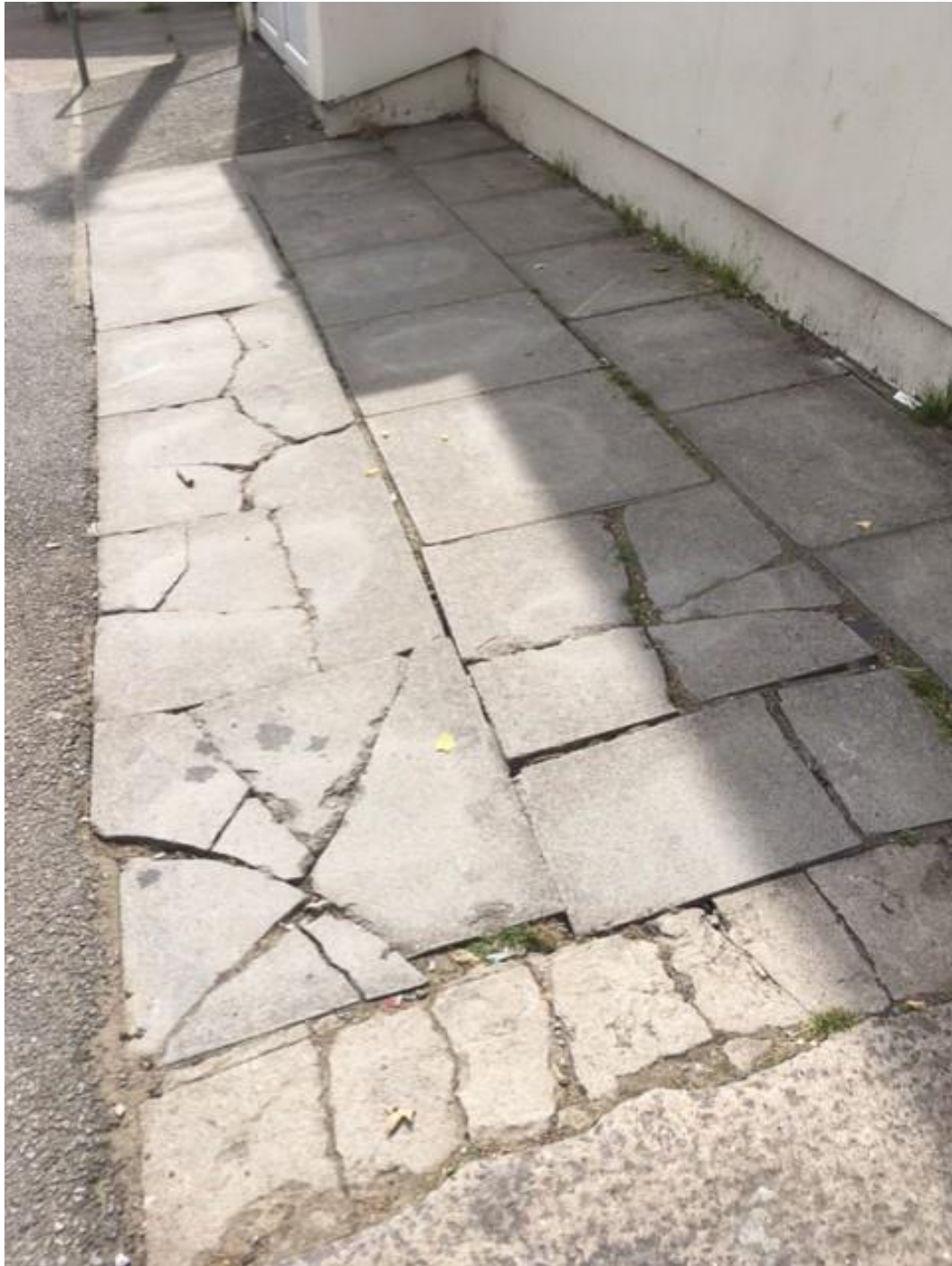
Cracked paving directly outside Llanharan Drop-in Centre in need of attention.
