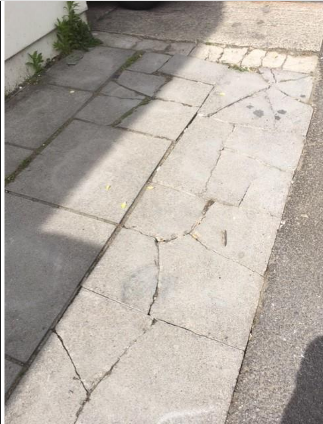
Please see raised paving, which could cause serious injury.
