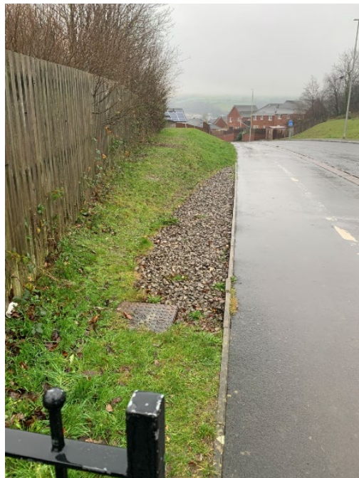
Picture 1a – Condition of ground along the ridge
