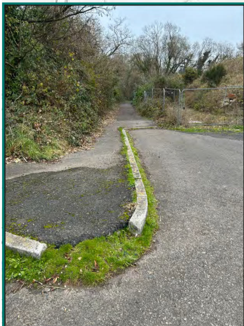
PHOTOGRAPH 2: ACCESS FROM NEARBY HOUSING ESTATE
