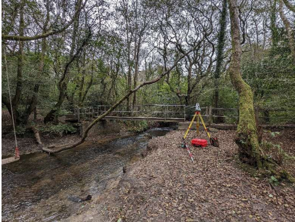
- Primary span of existing bridge (circa 9m)
