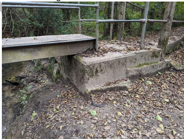
Existing concrete abutments -
