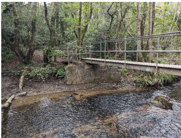
- Existing concrete abutments
